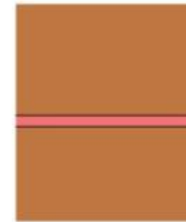
Original narrow red mortar joint in the decorative columns and panels to emphasize the brick detail and decrease the visual impact of the joint
