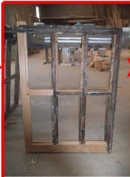
Window 15 during restoration, note as much original material as possible has been maintained
