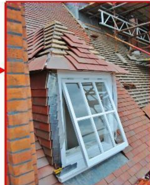
Window 15 after restoration and returned to its original location
