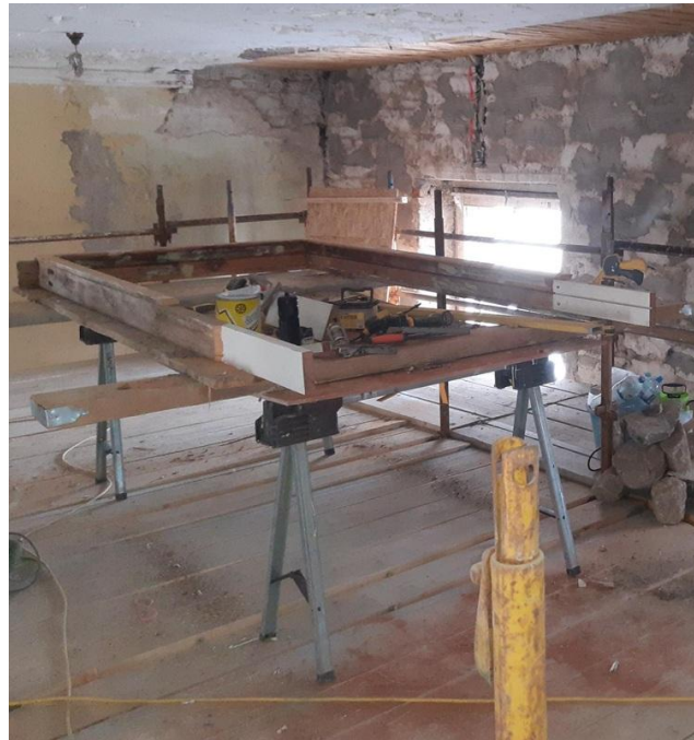
Window Repairs and Insulating Render
