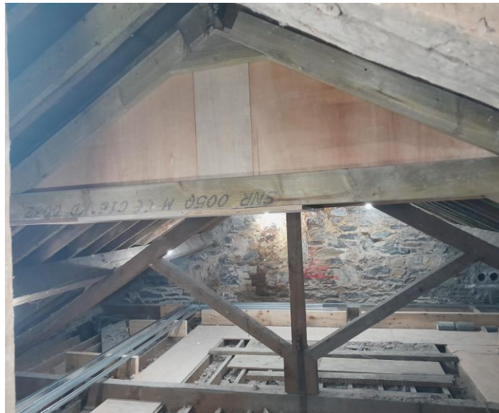
Accommodating Bat Roost in Attic Space
