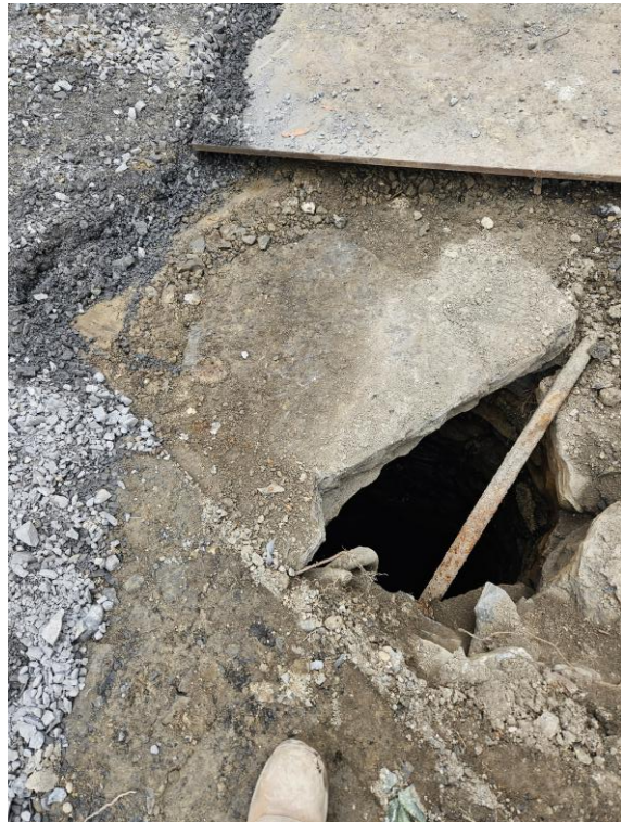
Well on Discovery – Covered with Flag Stone
