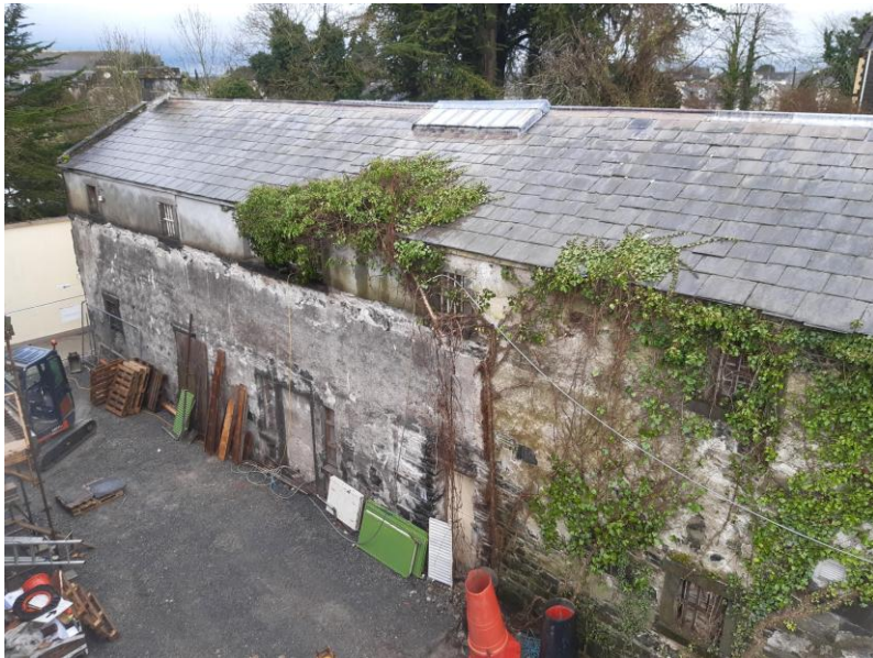
Demolition of Lean-to Extension on Adjacent Bridewell.
