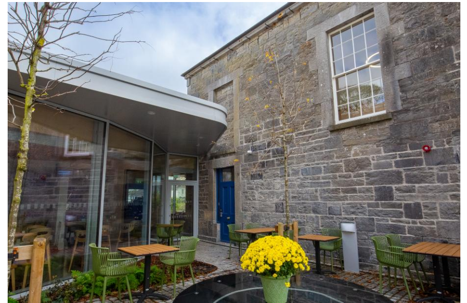
Downward Trajectory of External Lighting
