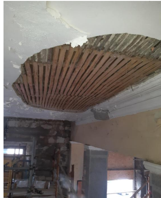
Decision to retain / repair existing lath and plaster ceilings
