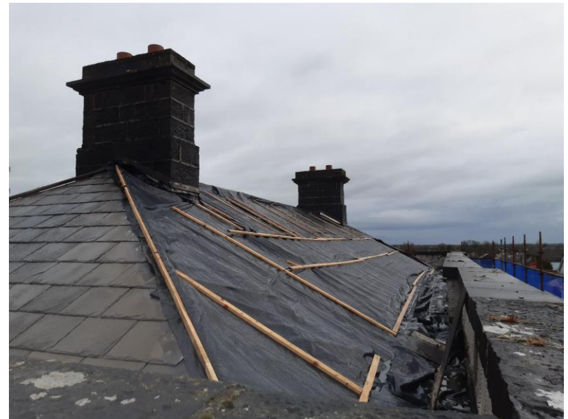
Temporary Covering of Exposed Roof
