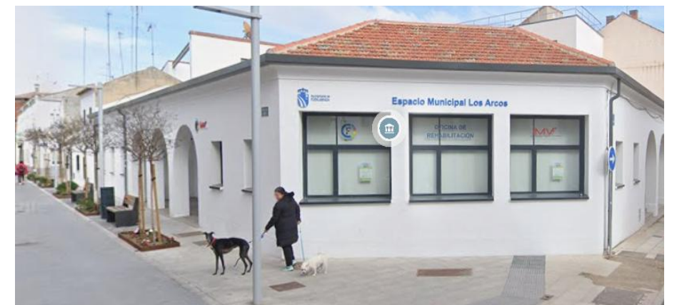
The first school in Fuenlabrada, rehabilitated during the implementation of the MILMA Project, co-funded by UIA.
