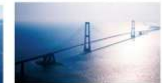
Great Belt Bridge (Denmark) 26,7 km
