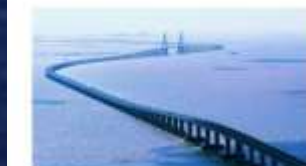
Jiaozhou Bay Bridge (China) 26,7 km
