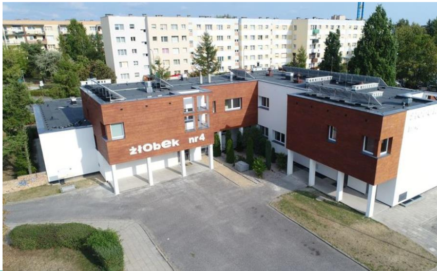
Comprehensive thermal modernization of public nurseries and kindergartens in the City of Kalisz
