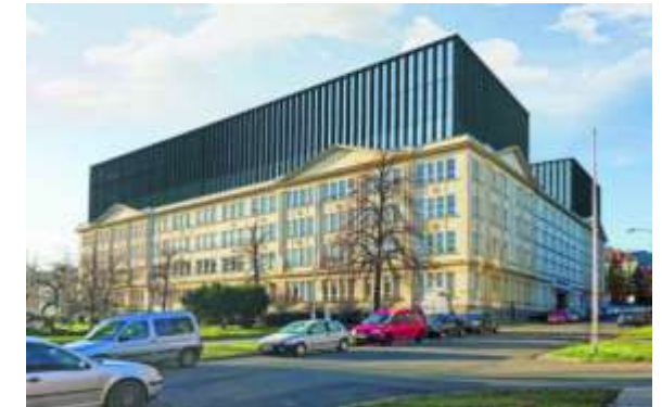
Czech Cybersecurity Center (CERIT Science Park II, Secondary School Čichnova Brno - technological center for cyber security)
